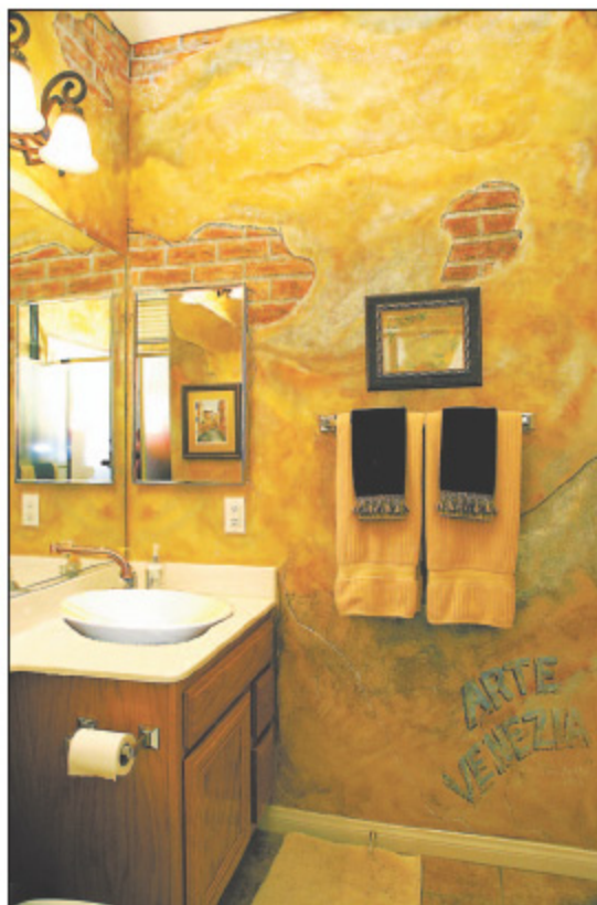
PHOTO COURTESY CHRIS SECKLER A faux Venetian plaster finish makes it appear as if once-covered bricks are being exposed by chipping plaster.
